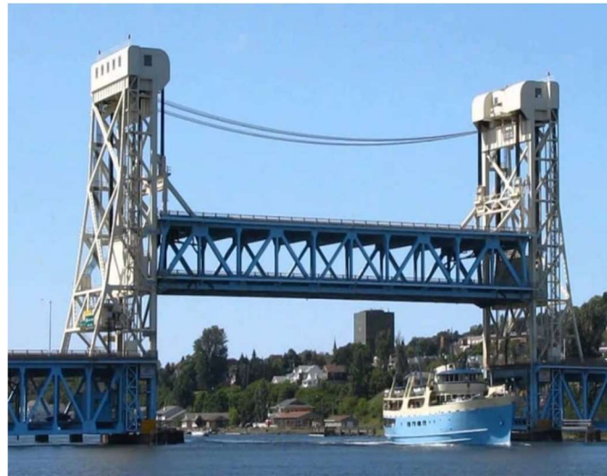
Figure 3.4.2.1.2 – Vertical Lifting Bridge [36]
