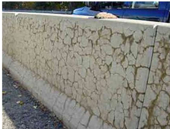
Figure 9.3.2.1.2 - Alkali Silica Reaction on Concrete Jersey Barrier [10]
