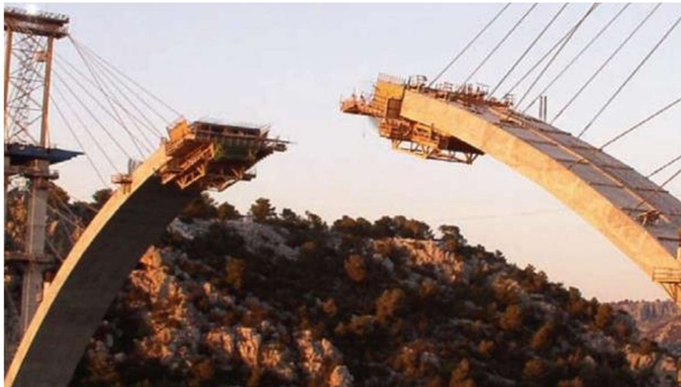
Figure 3.4.1.2.3 – Photo of construction of an arch bridge with travelling formwork method [30]
