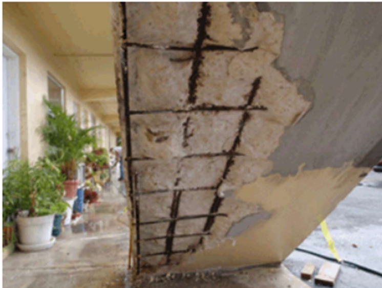
Figure 9.3.1.1.1 - Cracked Concrete Staircase due to Freeze and Thaw Cycles [7]
