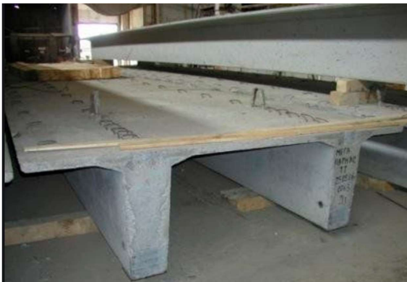
Figure 3.3.3.1 – Double T-Beam Cross Section [25]
