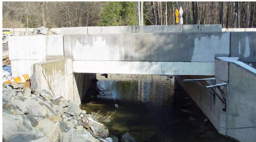
Figure 3.3.4.1 – Slab Bridge: [26]
