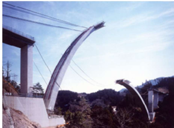
Figure 3.4.1.2.6 – Construction of an Arch Bridge by Lowering Method [33]
