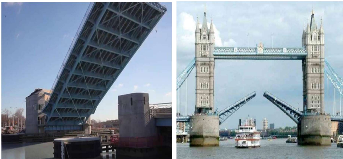
Figure 3.4.2.1.1 – Single and Double Leaf Bascule Bridge [36]
