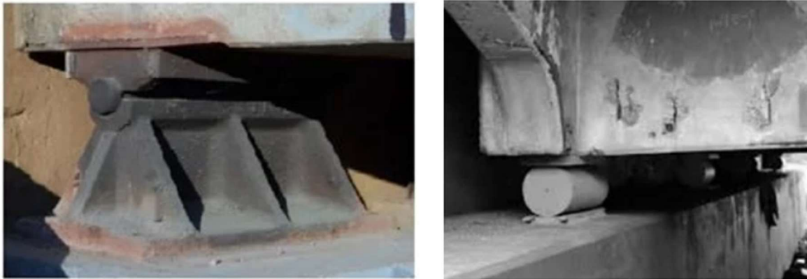
Figure 8.2.3.1 - Pin Bearing (Left) and Roller Bearing (Right) [2].
