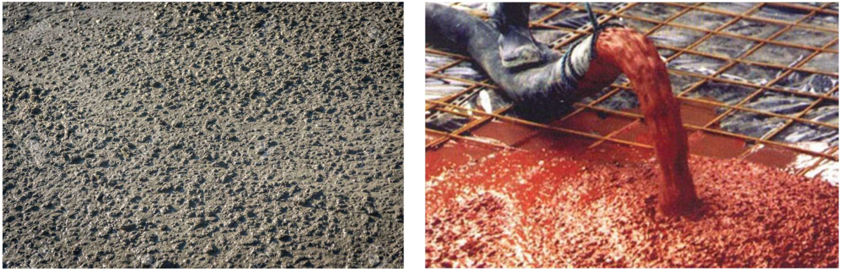
Figure 3.2.4.1 – (Left) Fresh Concrete and (Right) Colored Concrete due to admixtures (Photo from Prof Ahmet Topcu - Eskisehir University Lecture Notes)
