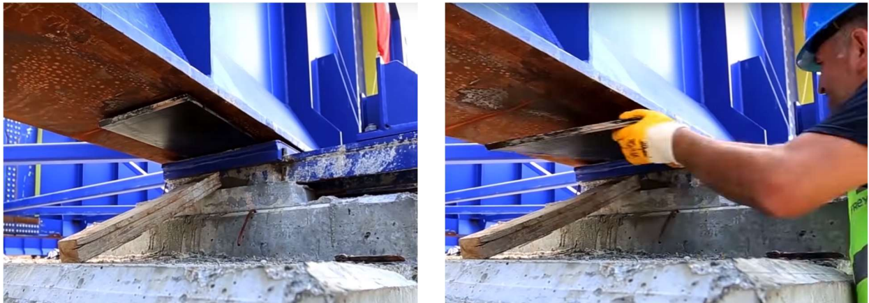
Figure 3.4.3.2.3 – Surface with less friction removal once bridge moves over support [46]
